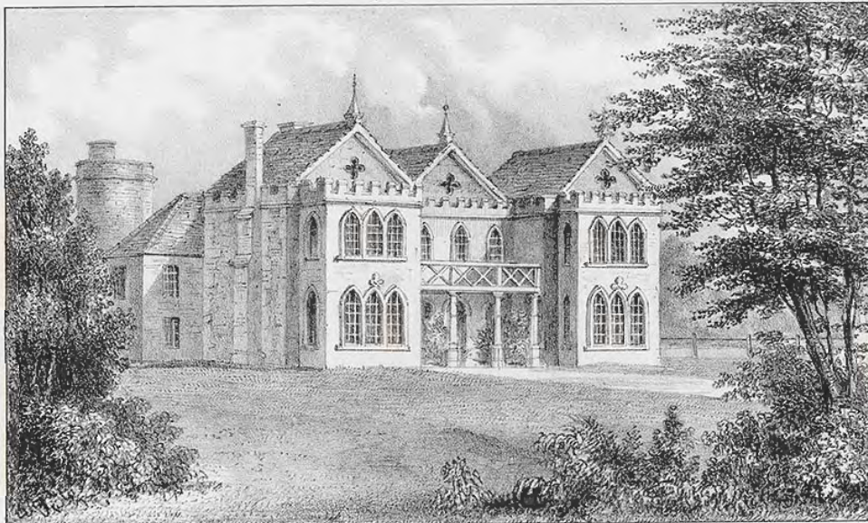
OLD WHADDON HALL. Formerly the Residence of Browne Willis Esq. "L.L.D."
