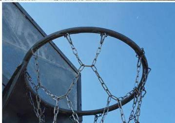
Finding: Inappropriate fittings have been used on the hoop Action: Replace with manufacturer spec hoop netting netting which is creating multiple finger entrapments in contravention of BS EN 15312
