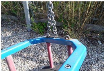
**Finding:** The swing seat connector is damaged and the chain is out of position
