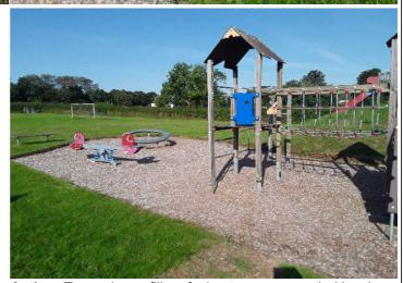
**Finding:** The depth of the loose fill surfacing is lower than the recommended depth specified in BS EN 1176; the free height of fall of the equipment is less than 2.0m and a minimum of 300mm depth should be provided (including an extra 100mm to allow for compaction and displacement as per BS EN 1176 Part 1 - Table 4)
