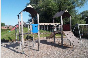
**Finding:** The height of the slide runout is in excess of 350mm and does not meet the requirements of BS EN 1176: Part 3
